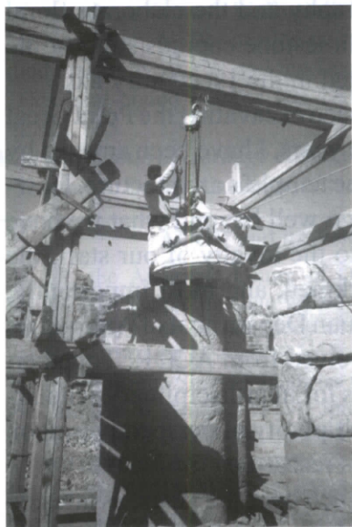
Restoration work; photo by Artemis Joukowsky
