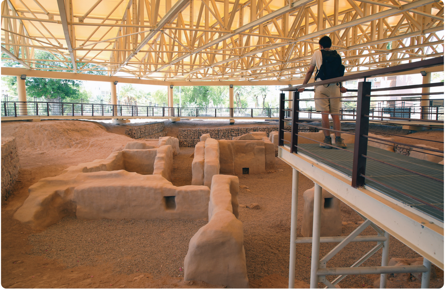
Above: A visitor on the walkway extension above the Aqaba Church, allowing a better view of the ruins, now sheltered from the elements. (Photo by Abraham Farajian.)
