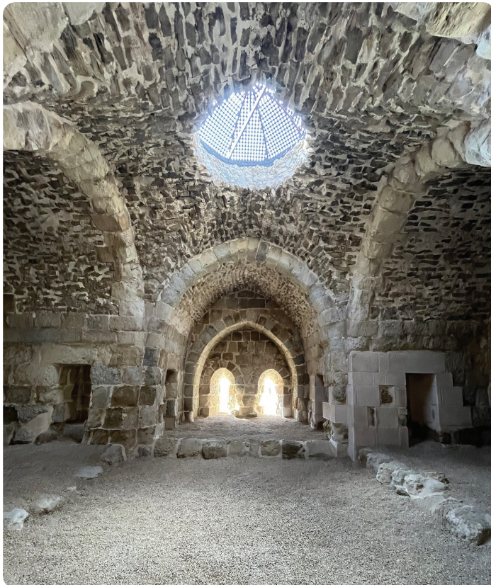
The interior renovation of the first level of Karak Castle's Tower 1. (Photo by P. P. Creasman.)
